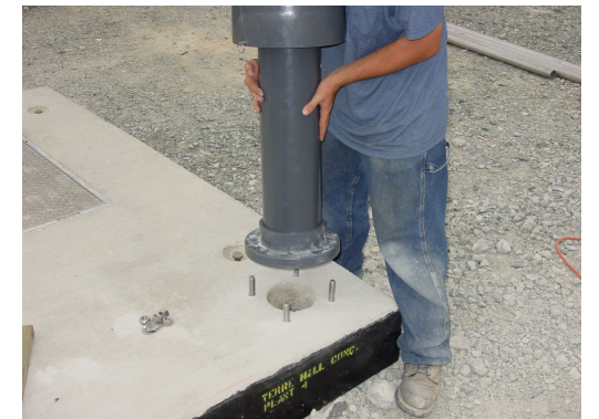
Simple mounting with SS wedge anchors.
